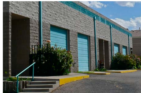
Large Office-Warehouse Building, Zoned C-3
