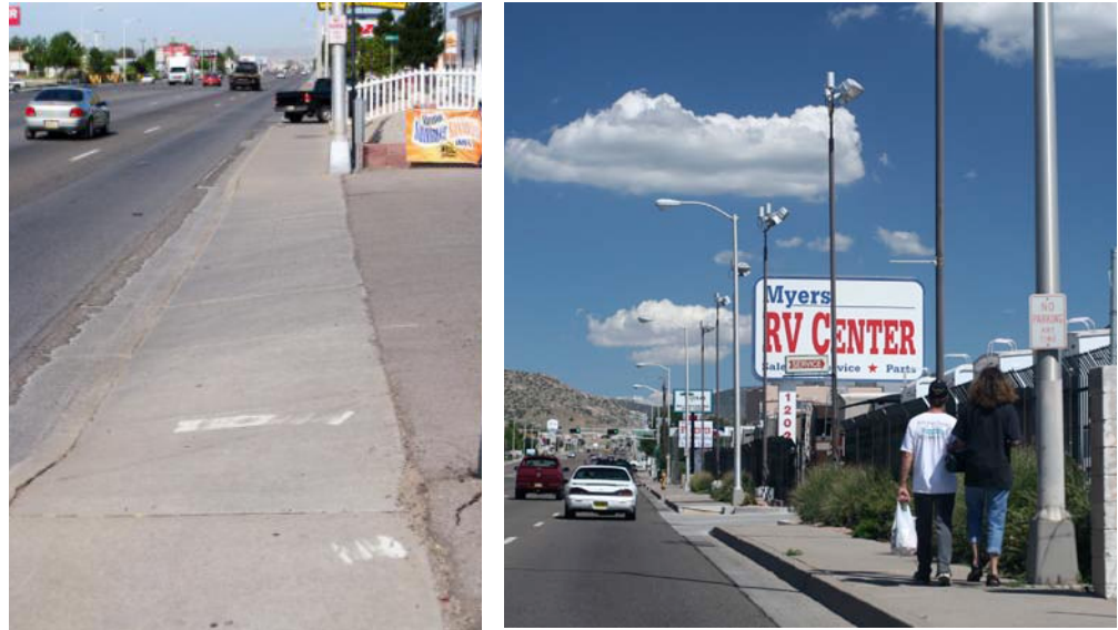
Figure 4.ee: Central Avenue Sidewalks
